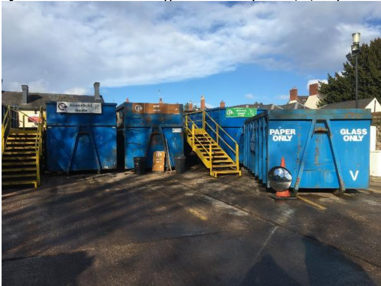
Figure 30: Containers Accessed via Stepped Metal Gantries (E.How 31/01/2019)
