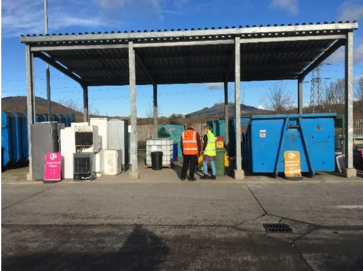
Figure 19: Central Covered Area
