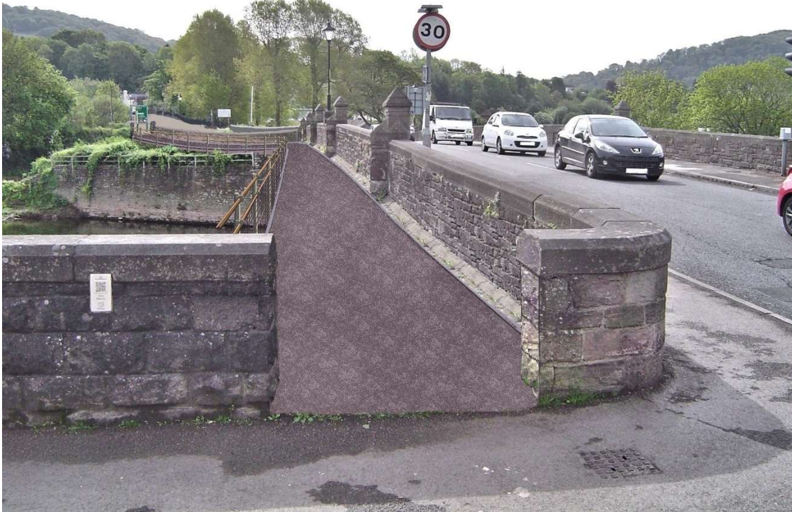
Plate 11 - Artists impression of Option II.I, one potential solution for Pedestrians and Cycles crossing the Wye
