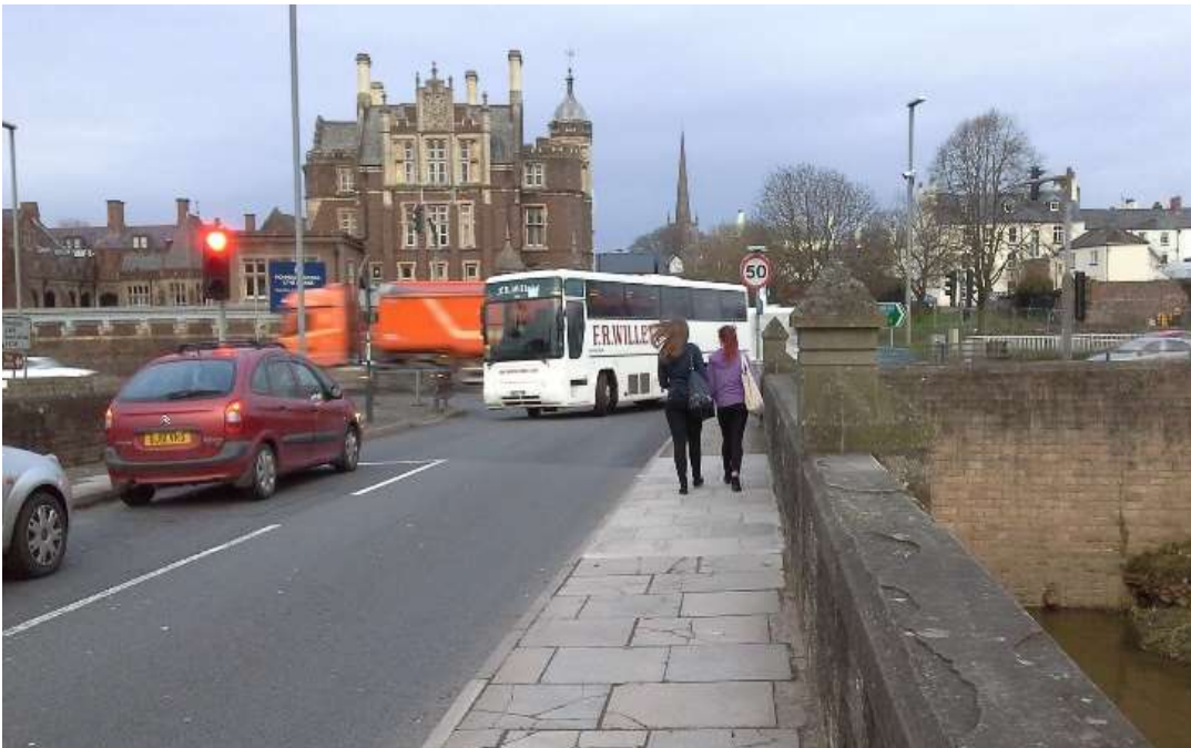
Plate 7 – View West along the Wye Bridge showing the impact of Public Service vehicles turning onto the bridge. This situation will worsen with the implementation of the Third Lane Scheme.
