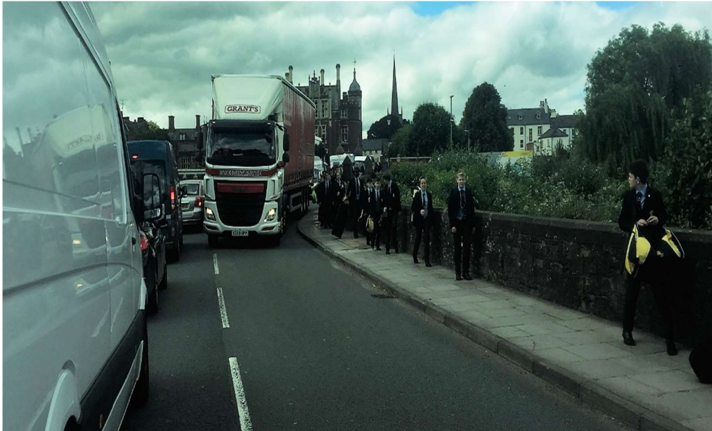
Plate 10 – Typical situation on the Wye Bridge with HGV's struggling to remain within the existing carriageways whilst large numbers of children are on the footpath. It is very evident in this photograph that pushchairs, wheelchairs and mobility scooters would inevitably result in children stepping into the road carriageway.
