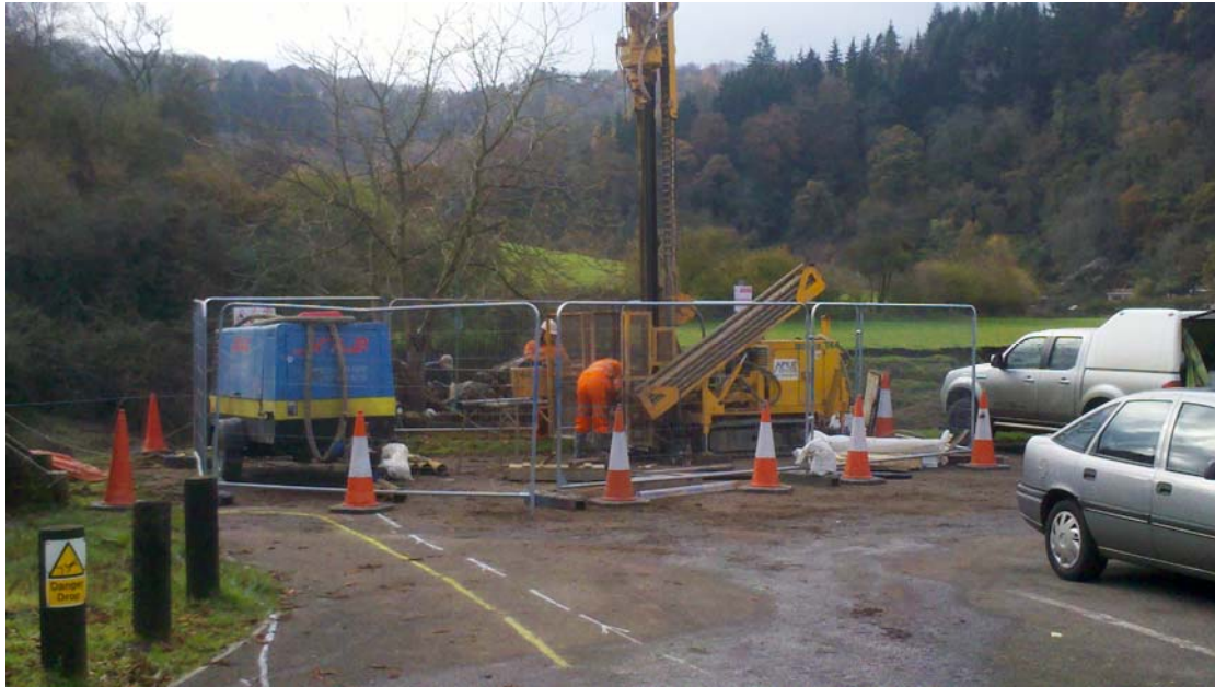
Drill rig in position in the car park
