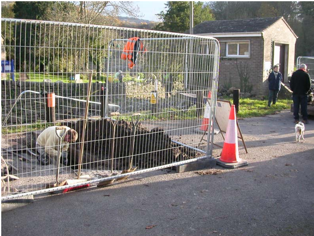
Trench in the car park to trace the services 'pipes' etc.
