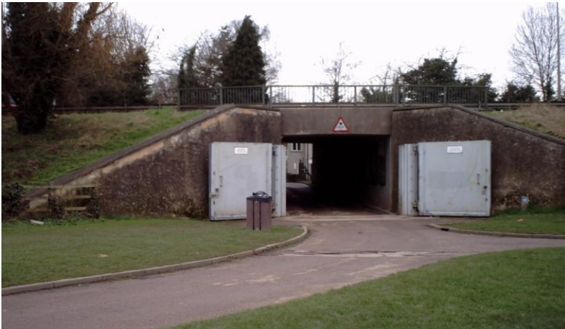
Figure 3-4 Flood gates on underpass
