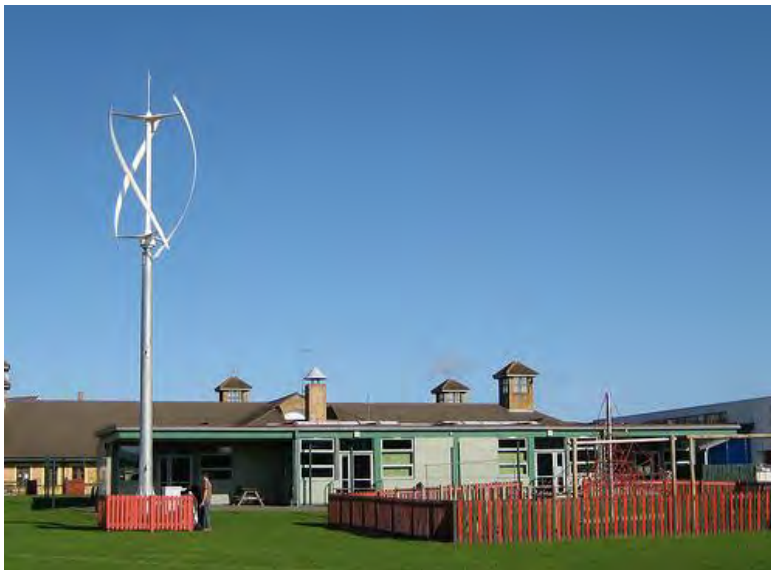
Vertical Axis wind turbine at Caroline Haslett School
