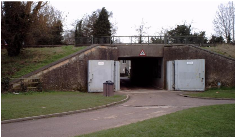
Figure 3-4 Flood gates on underpass
